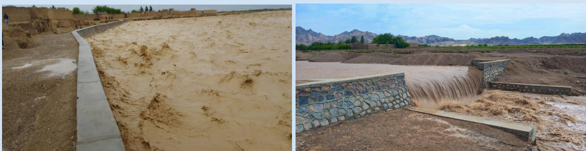
A protection wall constructed under AF1 in Zavol District, Herat Province, effectively protected nearby communities and their land from severe flood impacts, demonstrating its critical role in safeguarding lives, property, and local livelihoods (left) A check dam constructed under AF1 in Gulistan District, Farah Province, has played a vital role in protecting local communities from flood risks while also contributing to groundwater recharge (right)
