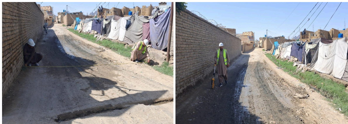
Site measurement during scoping for Arafat Plum Concrete Street with total length of 600 m, Gozar#3, District#3, Kandahar City in March 2026 @UNOPS
