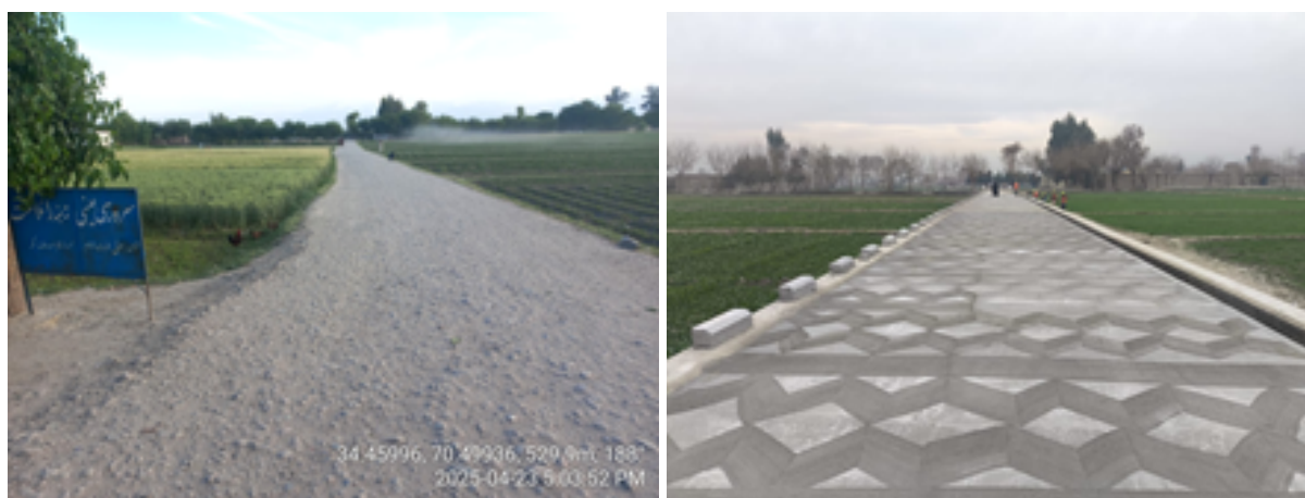
Before and after project photos of the digital pilot subproject, in Gozar #21, District #08 of Jalalabad City in February 2026 @UNOPS
