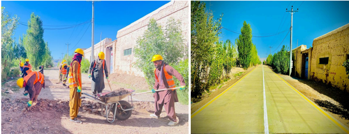
Upgrading of Samad khil and Zafaran khil villages street with plum concrete surface with a total length of 1235m in Gozar #15, District #2, Gardez city in March 2026 @UNOPS
