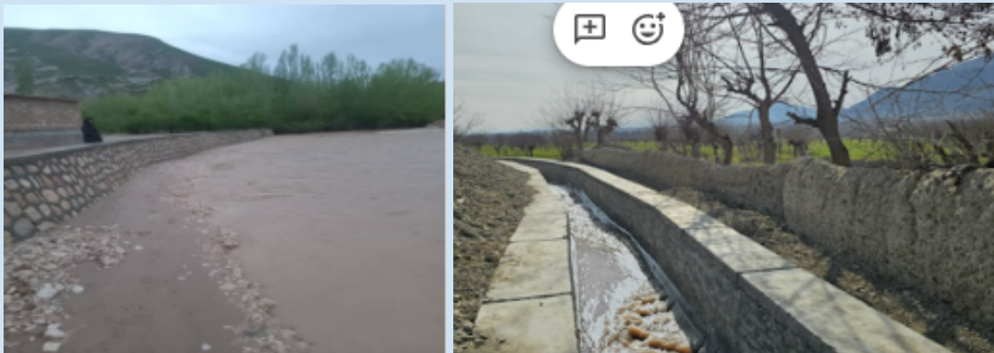
A protection wall constructed under the Parent Project (PP) in Bilchiragh District, Faryab Province, effectively safeguarded nearby communities and their land from flood impacts, demonstrating its importance in protecting lives, assets, and local livelihoods (left) .A canal constructed under AF1 in Nadir Shah Kot District, Khost Province, supports efficient water distribution for irrigation while protecting surrounding agricultural land, strengthening water management and enhancing local livelihoods (right)
