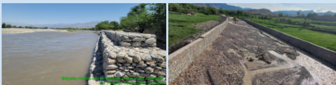
The retaining wall constructed under AF1 in Dasht-e-Archi, Kunduz Province, remains stable during heavy rainfall, effectively protecting adjacent road infrastructure and preventing erosion (left) A stone masonry protection wall constructed under AF1 in Gizab District, Urozgan Province, effectively protected the adjacent surrounding land from recent flood impacts (right)
