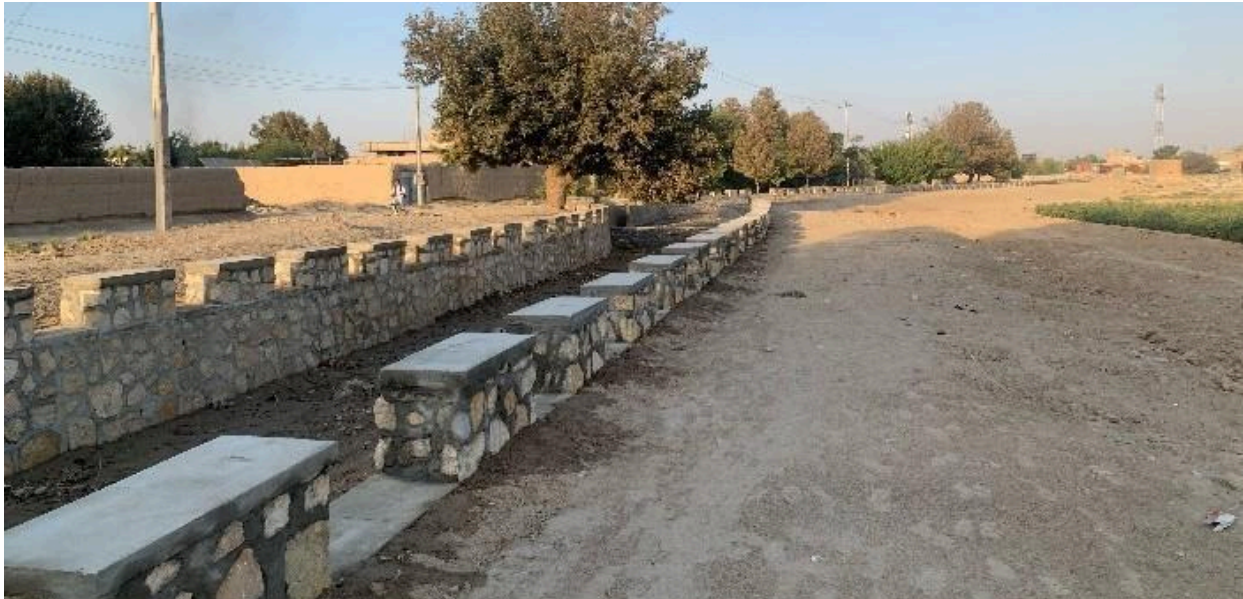
Storm drainage canal upgradation after completion of the DNP in Gozar #17, District #9, Mazar-e-Sharif City in March 2026 @UNOPS
